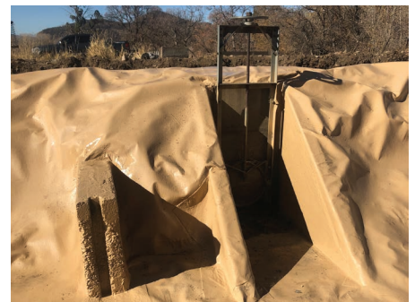
GROUNDGUARD liner sealed to the concrete structure will minimize erosion and seepage, preventing water loss.
