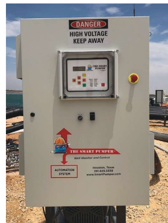
Smart Pumper is a universal platform (hybrid technology) that provides high-speed global connectivity with a processor that is used to support a multitude of applications to control and monitor anything through a customizable web-based interface from anywhere in the world. (Source: Direct Drivehead Inc.)
